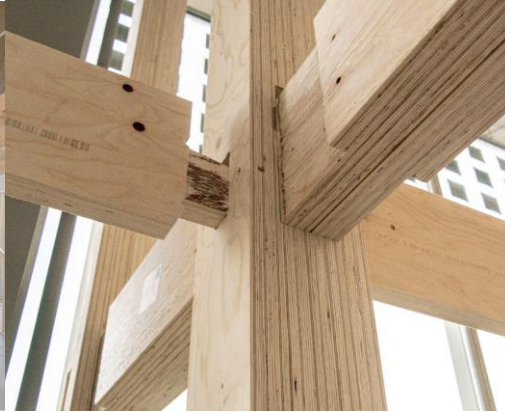
Hout-op-Hout verbindingen
